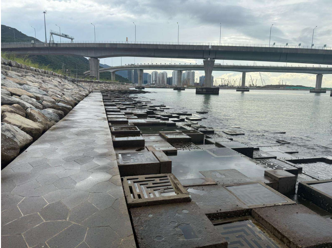
General View of Rocky Eco-shoreline
